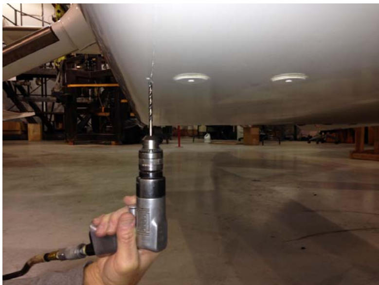
Figure 5-2: Finish Drilling Outside
